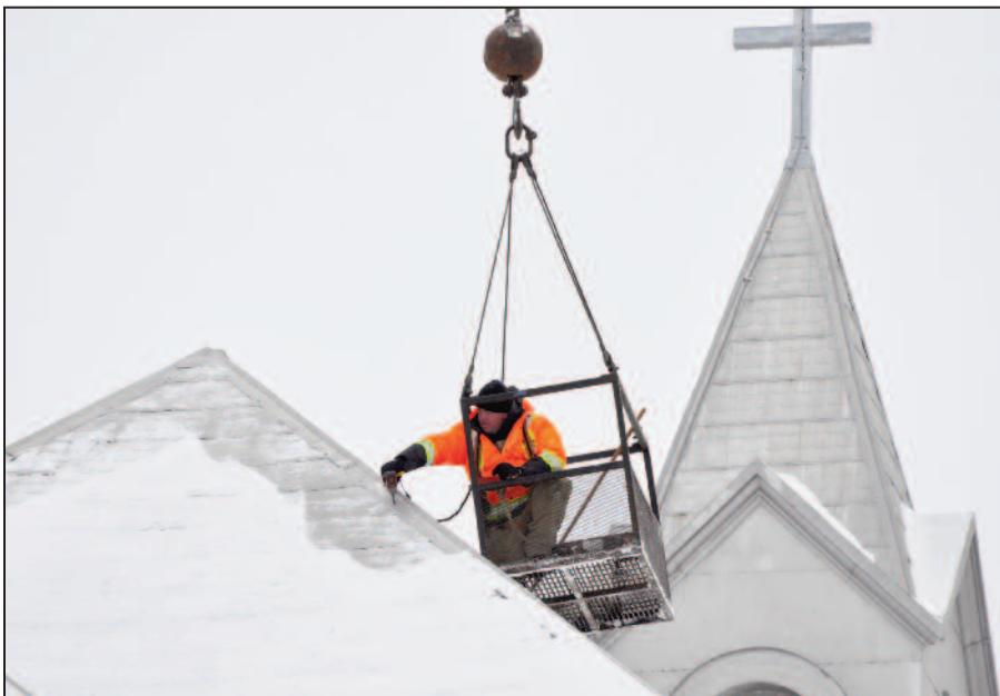
REPAIR COLLEGE ROOF – A crane supports a worker on the college roof during January when repairs were made to the roof.
