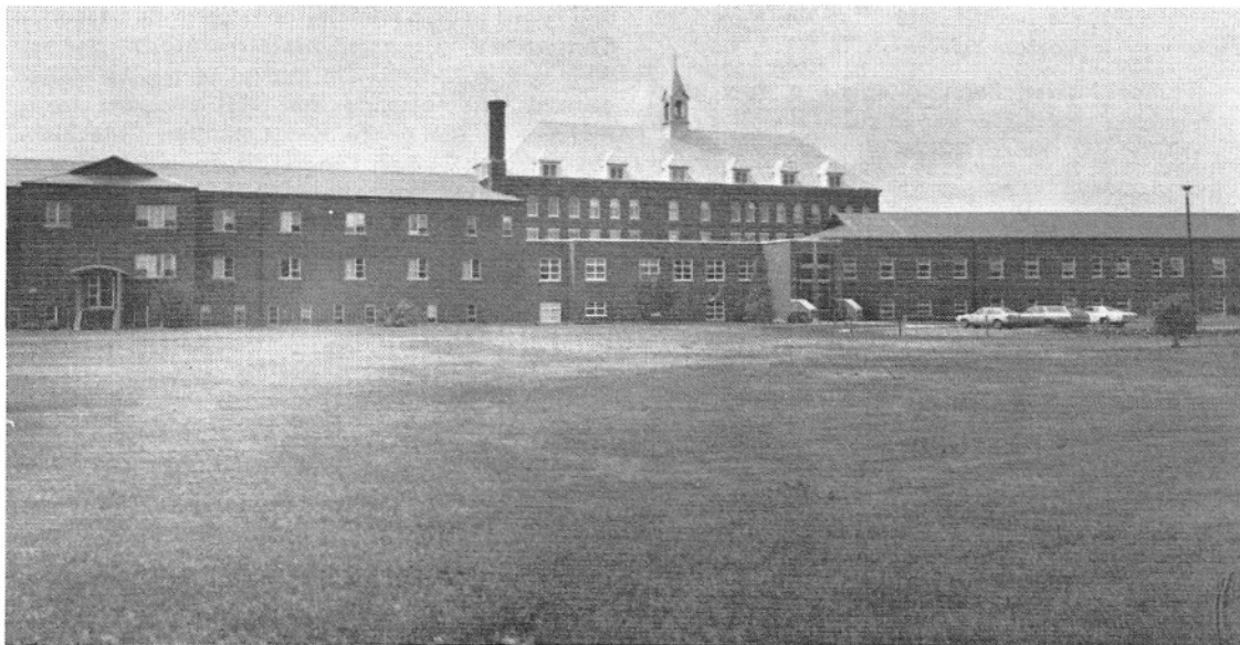
The recently completed metal peaked roofs give the abbey and Severin Hall a new look.
