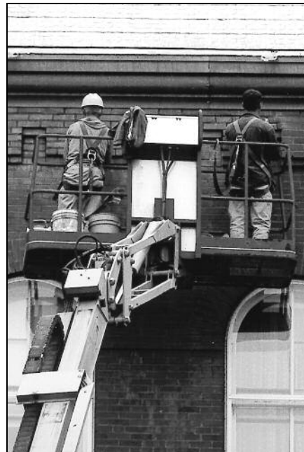
The repairing of the brick work of Michael Hall.
