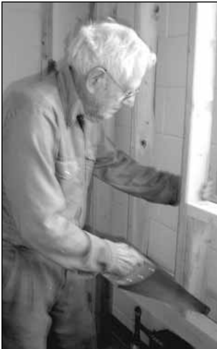
Br. Wolfgang prepares an inside wall for insulation in the abbey.
