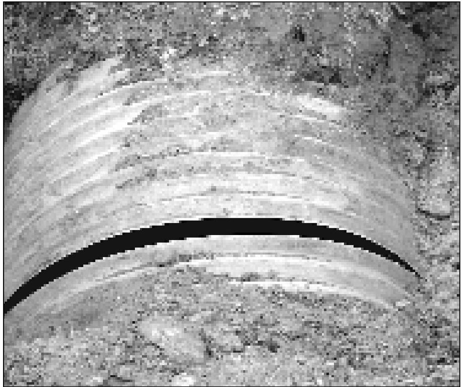
*This culvert on the abbey road to Muenster came apart on a seam during this spring's runoff.*
